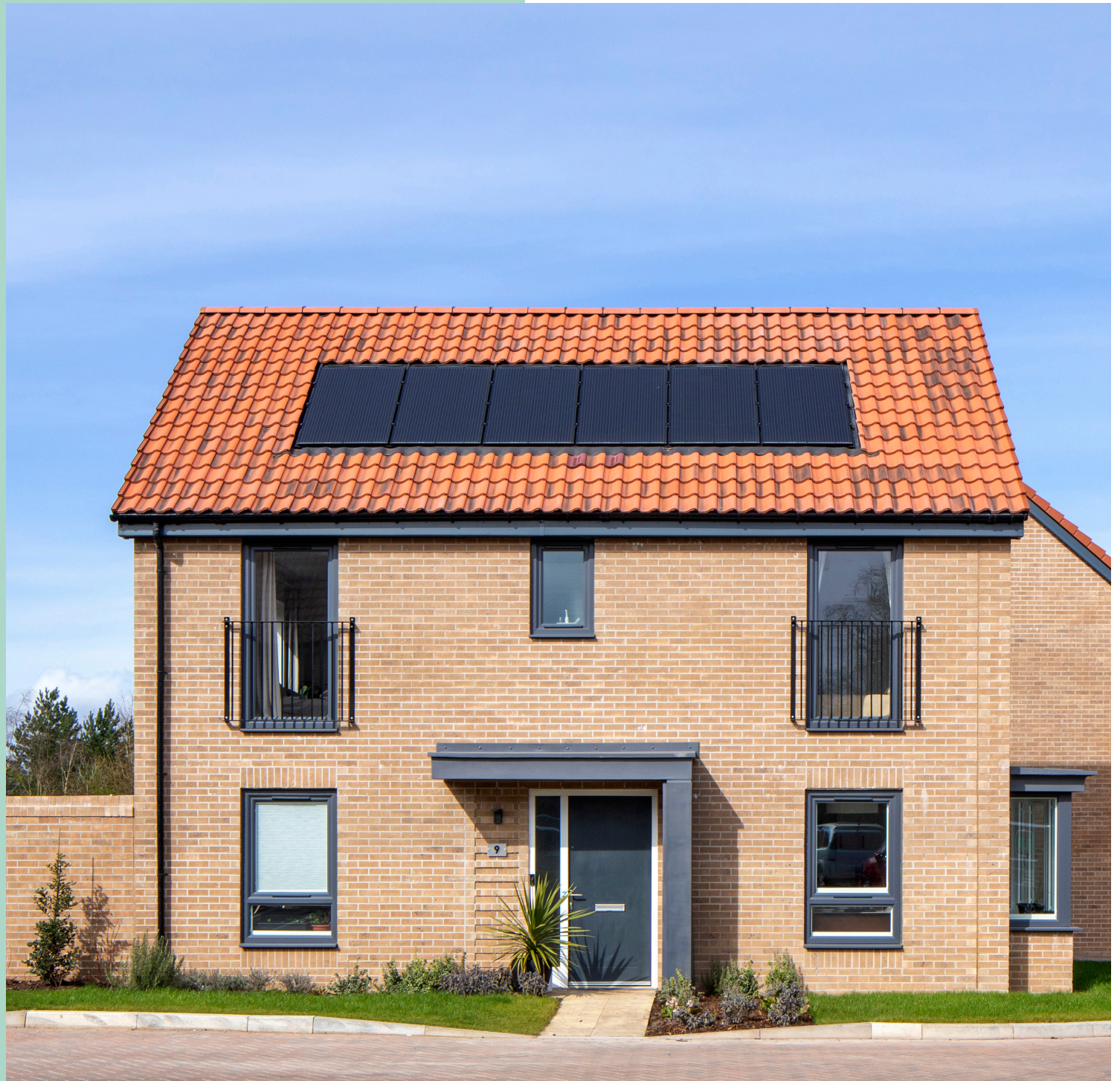
Above: Sustainable energy sources supply homes at Blackberry Hill, Bristol
